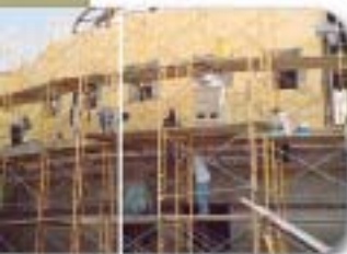
InsulBloc® adheres to CMU, poured concrete, primed steel, wood and most other construction materials.
